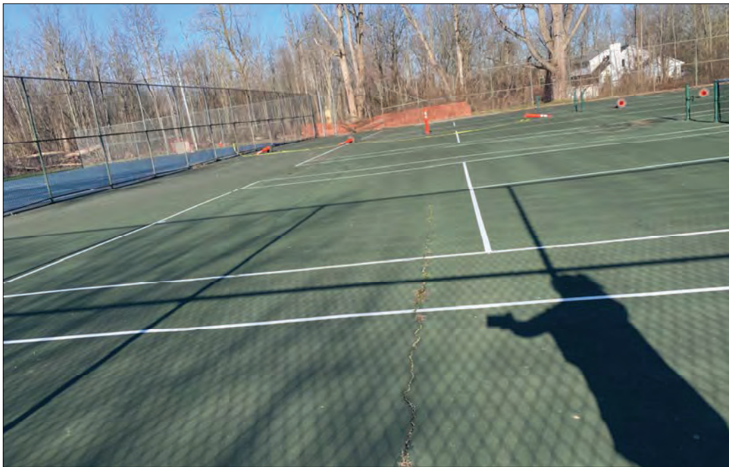
PHOTO 4 - EXISTING TENNIS COURT SURFACE
