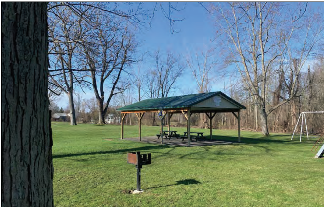
PHOTO 10 - EXISTING PAVILION AREA AND GRILL
