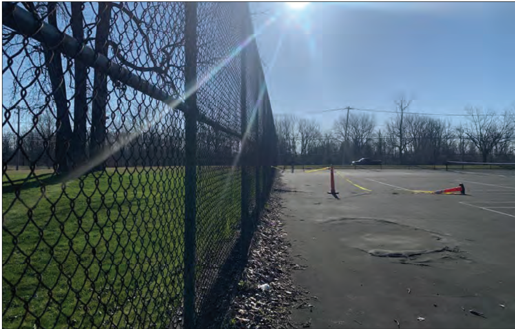
PHOTO 6 - EXISTING TENNIS COURT FENCING [NORTH SIDE]
