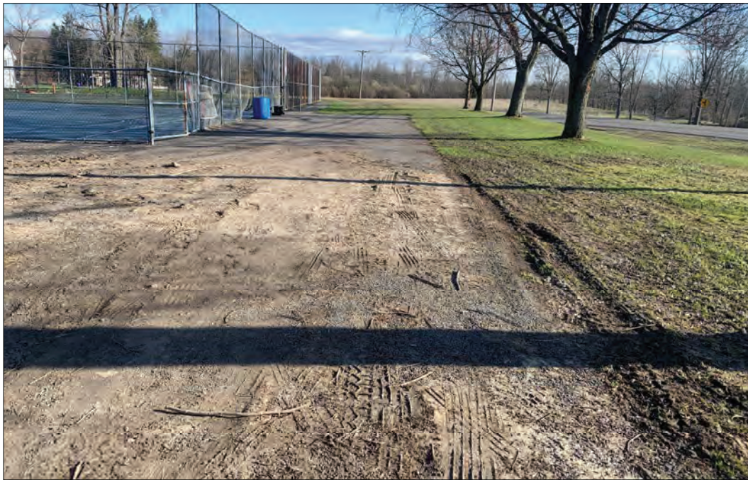
PHOTO 1 - EXISTING ASPHALT PAVEMENT AND WALKWAY AREA NEAR SPORTS COURTS
