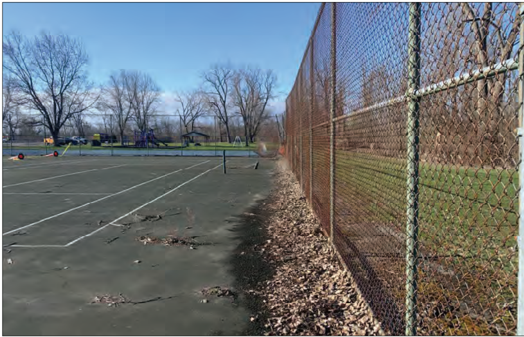
PHOTO 5 - EXISTING TENNIS COURT FENCING [WEST SIDE]
