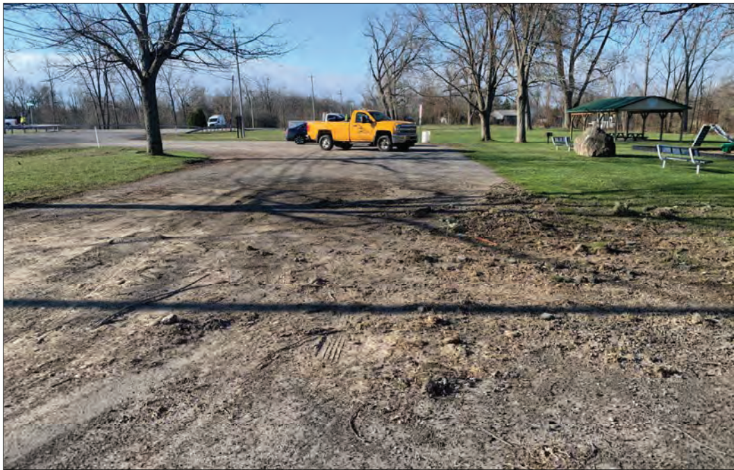
PHOTO 7 - EXISTING GRAVEL PARKING LOT
