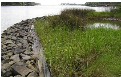
Stone breakwaters to protect plants and deflect debris.
