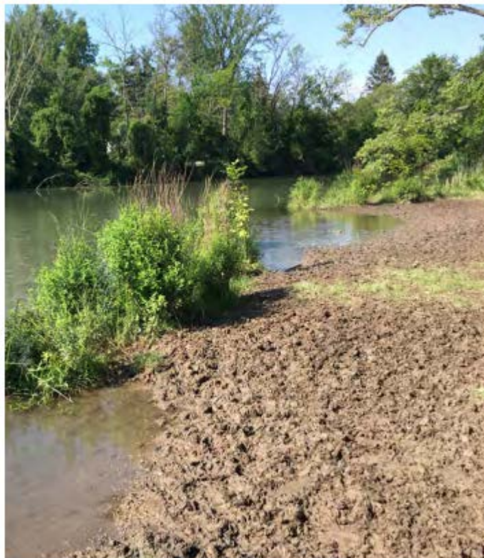
Poor shoreline conditions at Ellicott Island Bark Park
