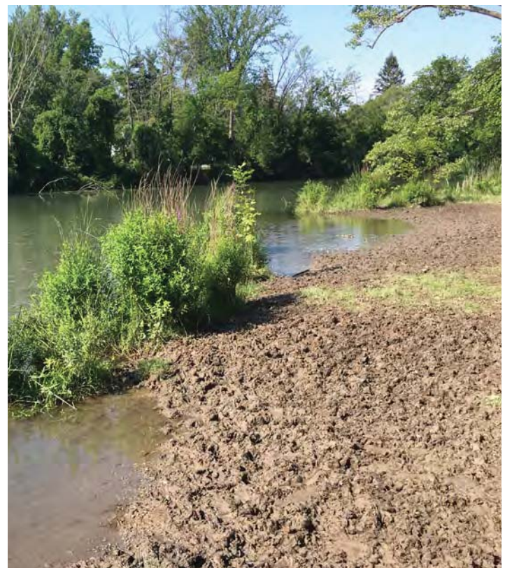
Poor shoreline conditions at Ellicott Island Bark Park
