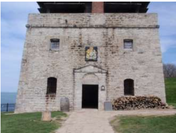
North Redoubt, Southwest Face, Overall View.
