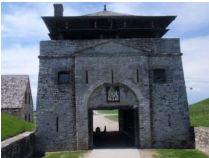
South Redoubt, Southeast Face, Overall View
