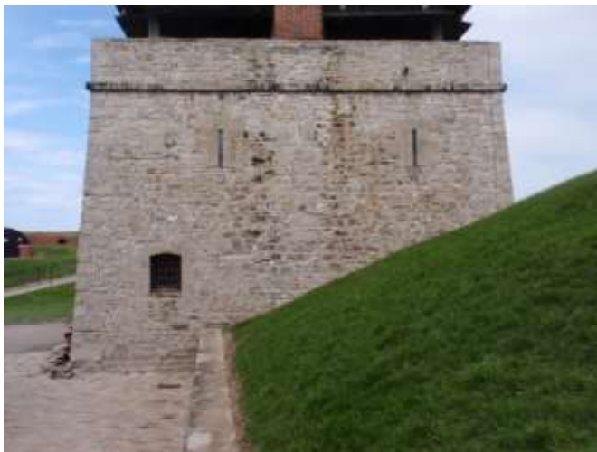
South Redoubt, Southwest Face, Overall View
