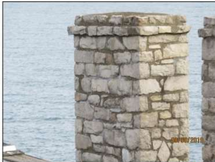
Chimney #1- Southwest sides
