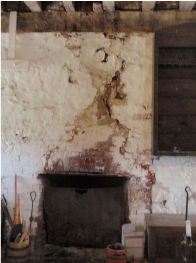
S4- South Redoubt first floor interior 05 west wall
