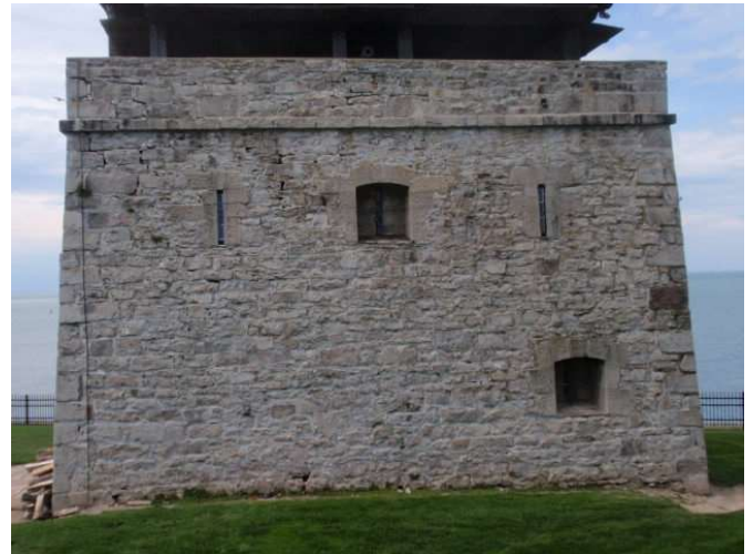
North Redoubt, Southeast Face, Overall View
