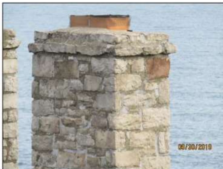
Chimney #2 - Open Clay tile flues
