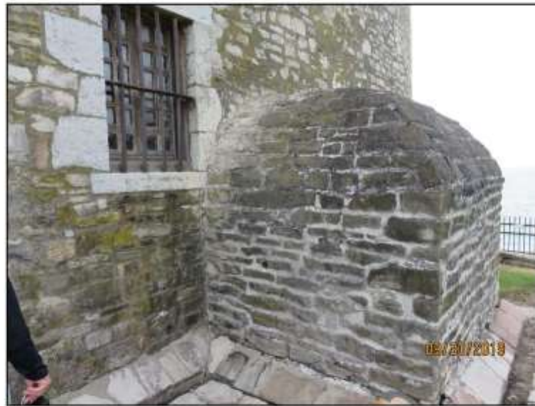
Chimney 2 base south elevation
