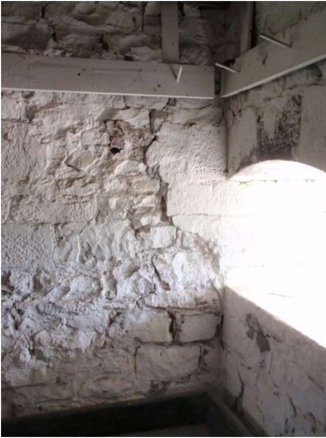
S5- South Redoubt first floor interior 07 northwest corner
