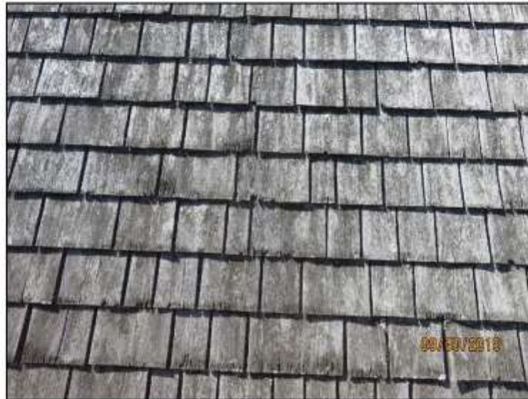
Typical condition of roof shingles
