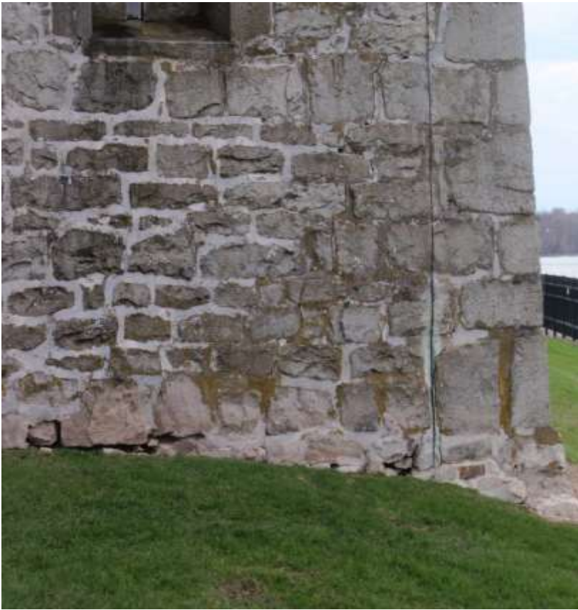
N1- East facing detail 07, foundation 05
