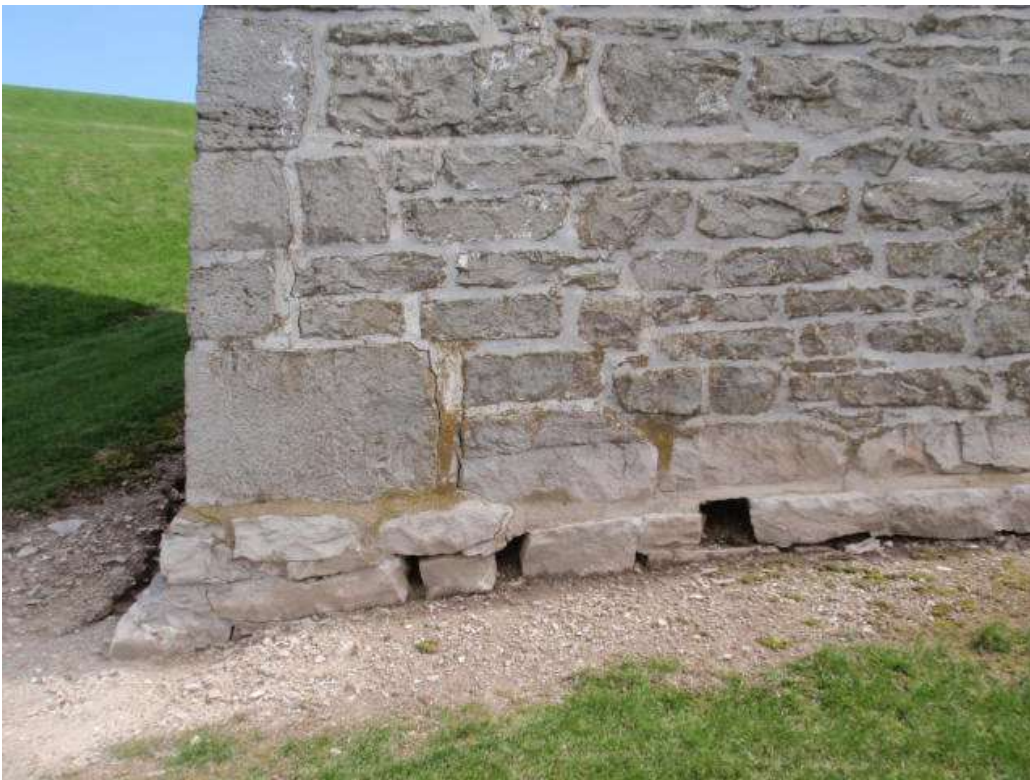
N6- North Redoubt North foundation 01 lower left corner
