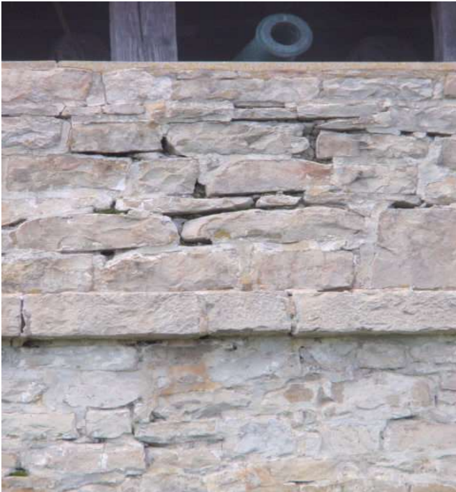
N8- North Redoubt South facing detail upper middle
