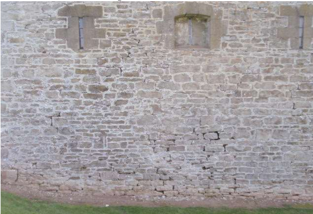
S2- South Redoubt east facing detail 02
