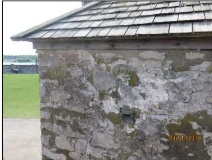
Scupper at third floor level
