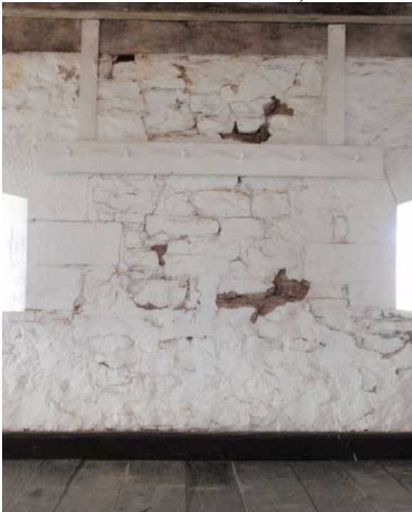
N4- North Redoubt interior 06, first floor South wall
