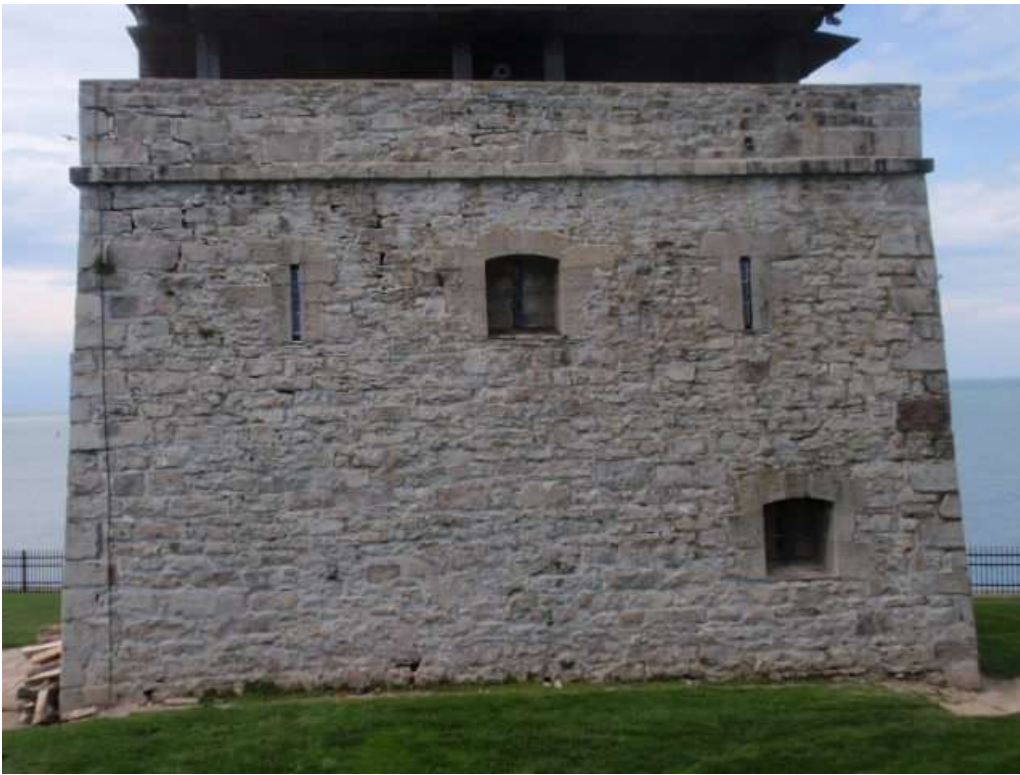
N7- North Redoubt South facing
