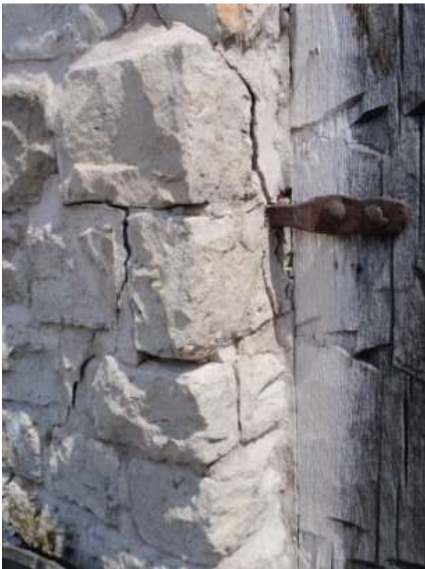
S8- South Redoubt north facing detail 03
