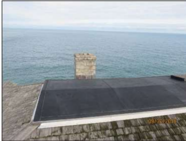
Chimney #7 adjacent to Modern EPDM roof
