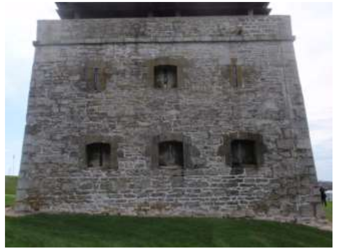
North Redoubt, Northeast Face, Overall View
