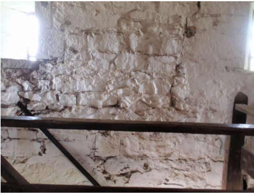
S7- South Redoubt first floor interior 10 east wall
