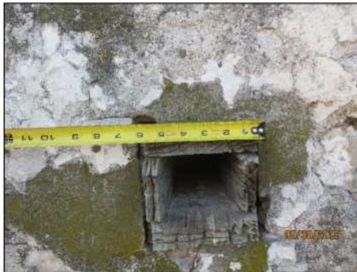
Close up of scupper
