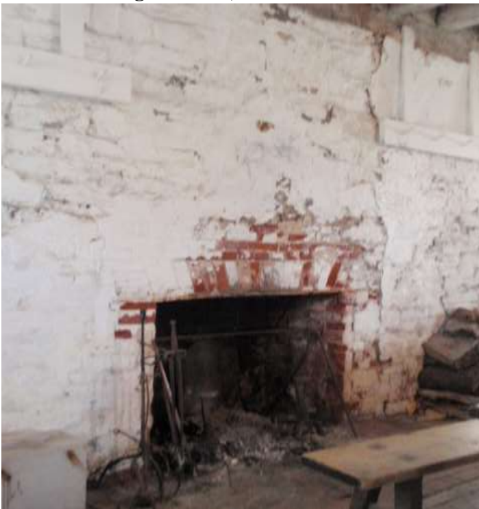
N2 – North Redoubt interior 01, first floor West wall
