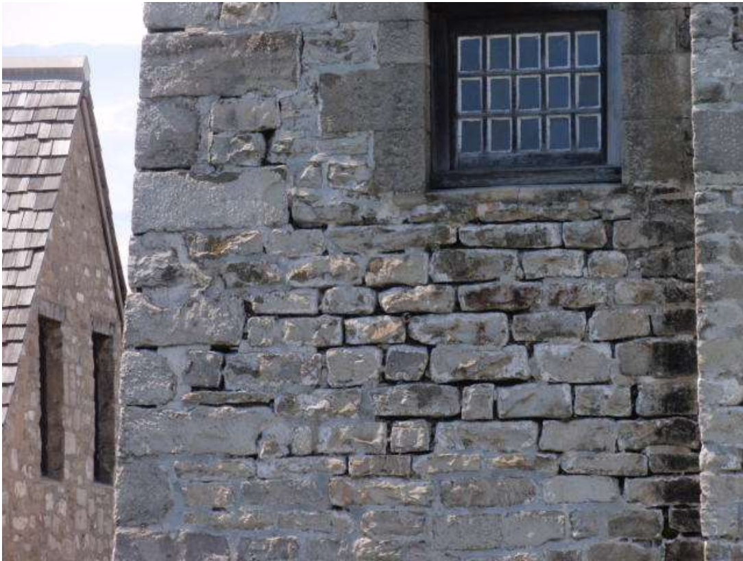
S9- South Redoubt south facing detail 02
