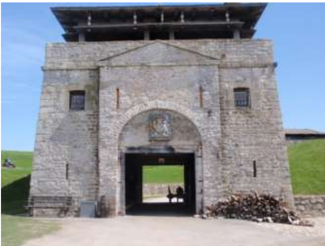
South Redoubt, Northwest Face, Overall View
