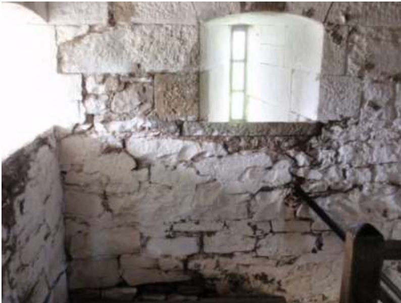
S6- South Redoubt first floor interior 08 northeast corner
