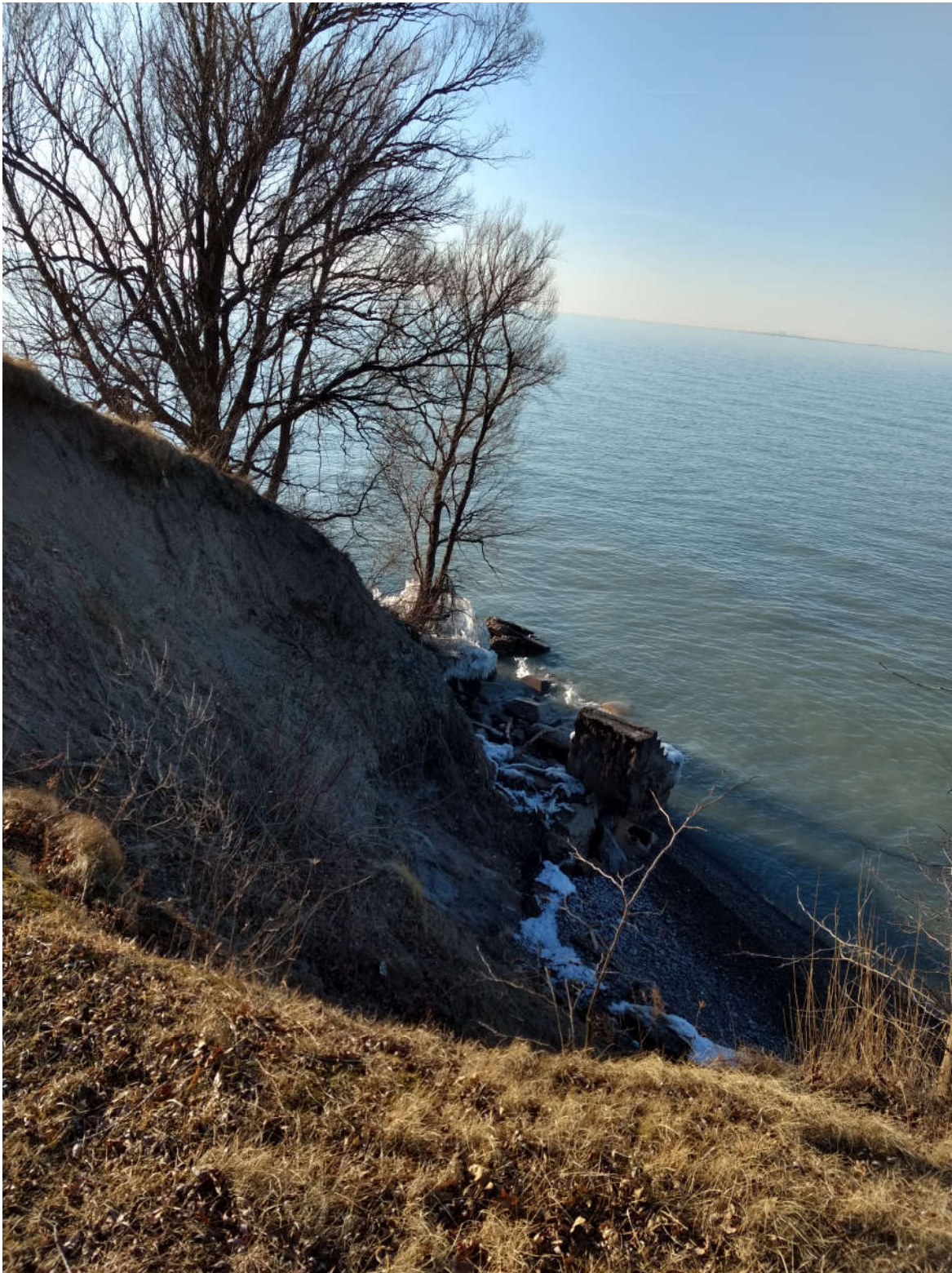
Photo #2: View of proposed shoreline stabilization area, west end.
