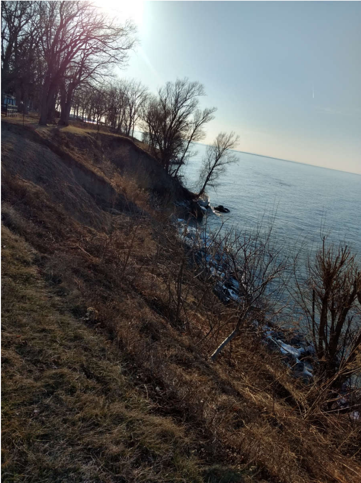
Photo #1: View of proposed shoreline stabilization area, looking west.
