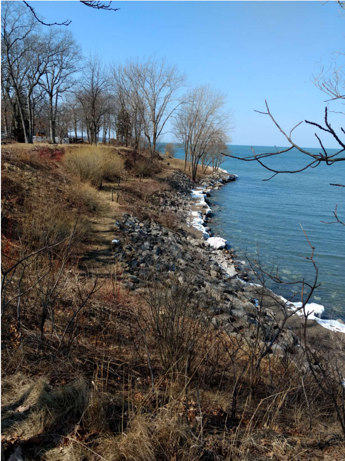
Photo #4: View of adjacent (west) stabilized shoreline.
